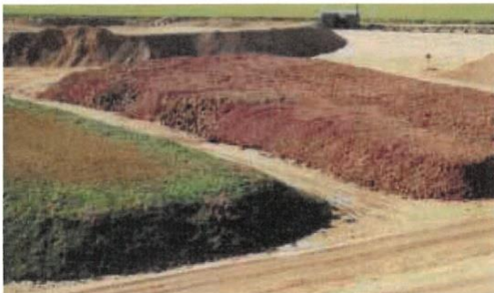
Clearly defined stockpiling of different soil materials
