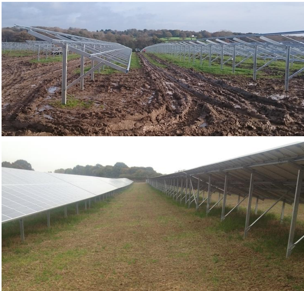
Inserts 26 and 27: Inter-row Ground Restoration
